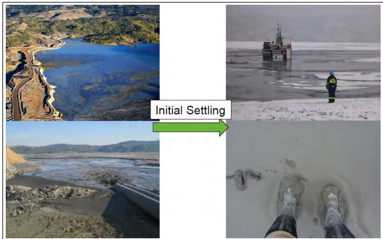
Figure 4 Illustration of Initial Settling of Tailings at the YDTI
